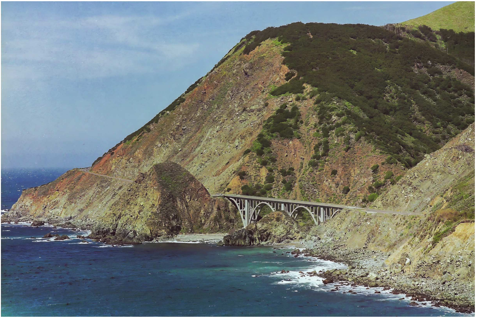
An engineering challenge on Route 1
