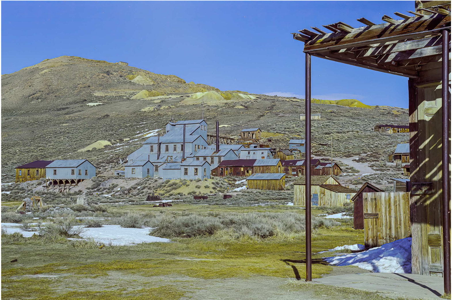
Day 7 - Abandoned mine workings at Bodie
